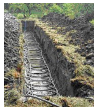
Figure 4: GSHP pipework
